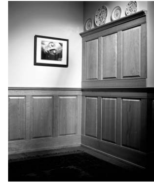
Outside Corner With Miter Joint
