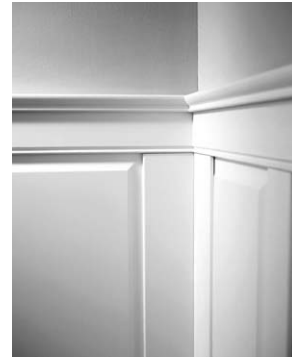
Inside Corner with Miter or Cope Joint
